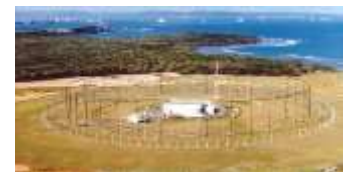
Circularly Disposed Antenna Array (CDAA) built for HF monitoring & direction finding. Wahiawa, HI
