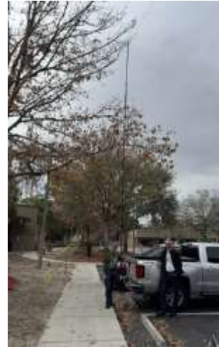
(L) This is a temporary HF antenna set up in the front of the EOC resulting from a damaged coaxial cable to the OCF & End Fed HF antennas in back.
