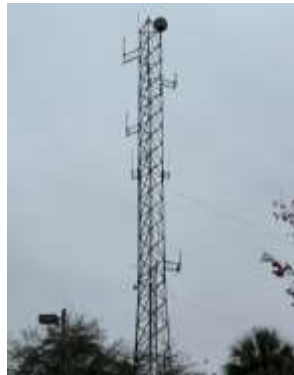
This 150 ft tower supports 2 Meter & 70 cm antennas.
