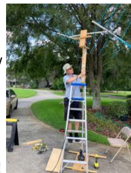
Jeff Capehart W4UFL working on a "Satellite Tower"
