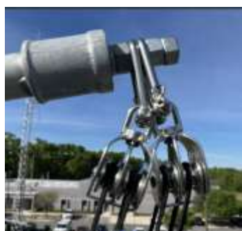
L1) The 15-year-old lift pole needed help. (L2) A view of the old lift pole shows the OCF transformer was permanently mounted preventing easy maintenance access. Center – The new hurricane rated tower was designed using pulleys for accessing the existing (and future) HF antenna hardware at any time. (R1) County employee installing the new hardware. (R2) Finished!
