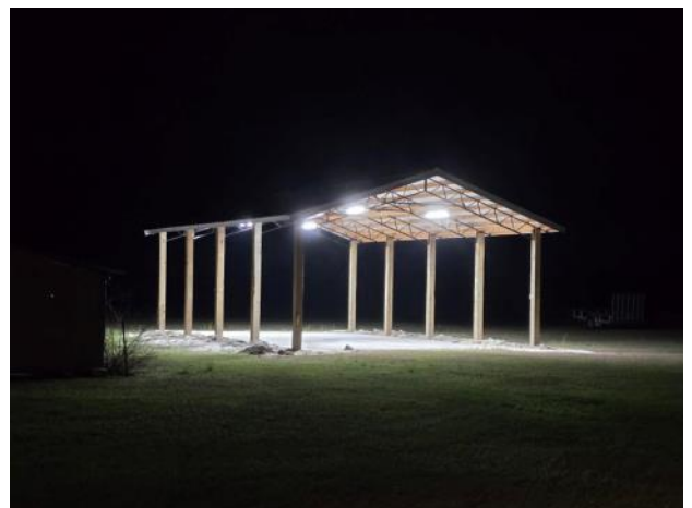
Four Harbor Freight shop lights light up the area under the roof and out at least fifty feet onto the lawn.
