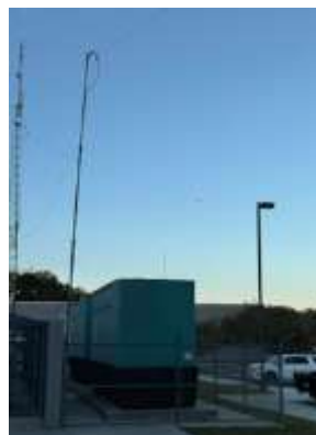
New Location of the HF Tower Supporting the OCF Antenna
