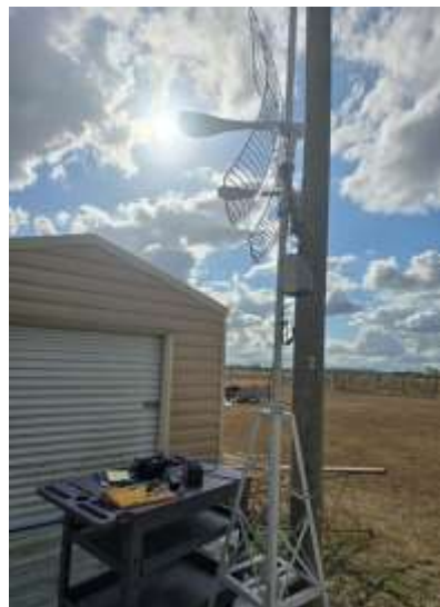
Grid dishes on 1296 and 2304 MHz at roof level.
