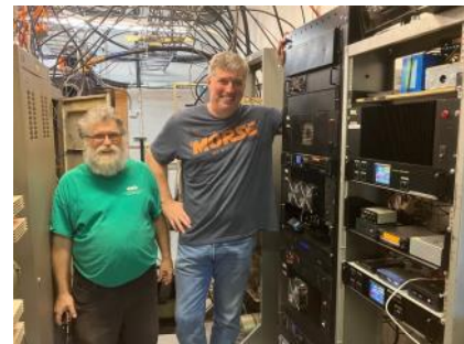
Jim Carr KC4MHH (L) and Jon Simonds KC4NWK (R) standing beside some of the impressive repeater bank @ TV-20 receiving tower. They generously make multiple repeaters available for disaster service.
