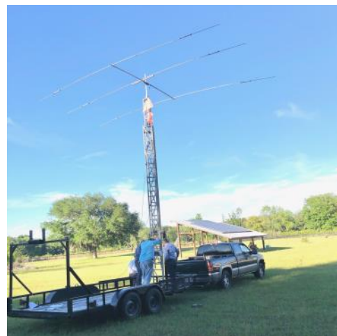
TA-33Jr on nested tower. We don't have guy lines yet. Or a winch, either! We "walk" it up and down. 2-3 people make it easy.
