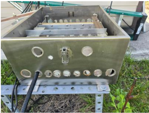
Here is a top view. Additional lightning arrestors are going to be installed for 75 Ohm antennas, Ethernet and control cables. The hinged lid closes like a coffin.
