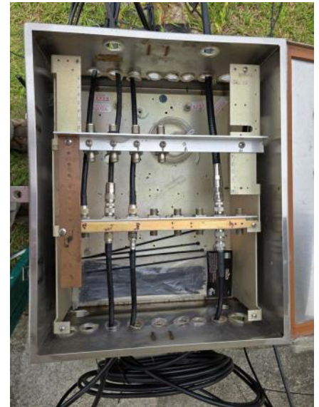
Here is a top view. Additional lightning arrestors are going to be installed for 75 Ohm antennas, Ethernet and control cables. The hinged lid closes like a coffin.
