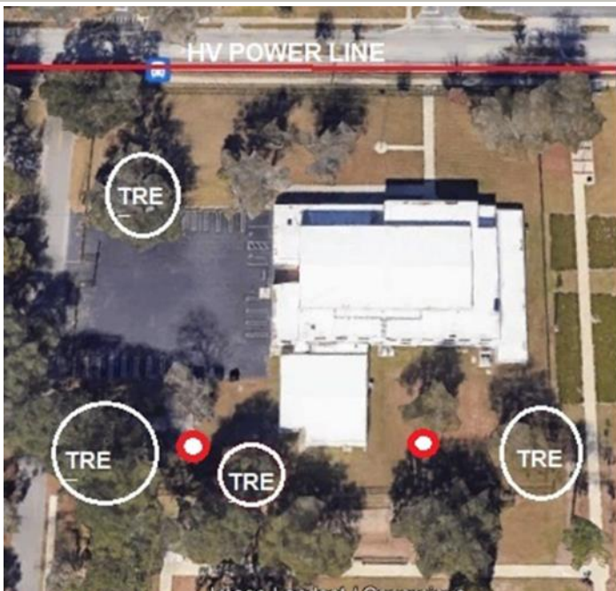
Figure 4: Baseline noise measurements locations #1 (left) and #2 (right) shown in satellite view. A High Voltage power line runs east-west on the street north of the building, and the power transformers powering building are centered along the east wall of the building. TRE = tree.
