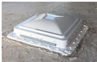
New RV Vent installed to stop one of Gordon's pesky leaks!
