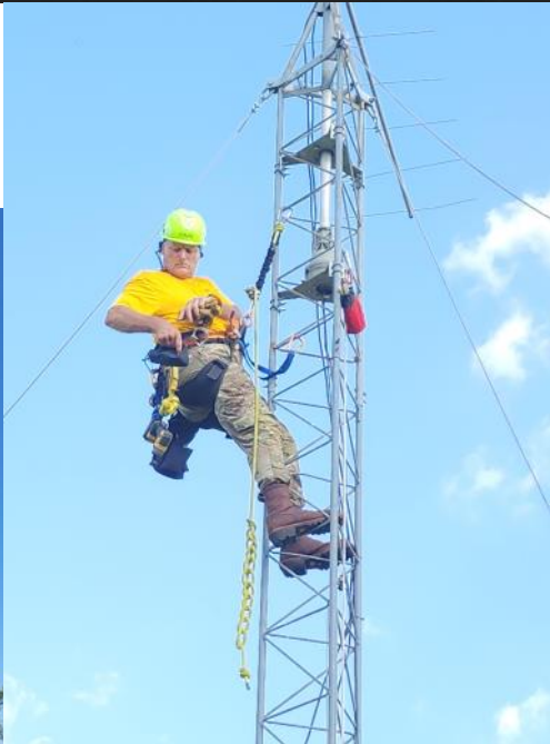
Left & Below—Mark installing the G7-144 antenna
