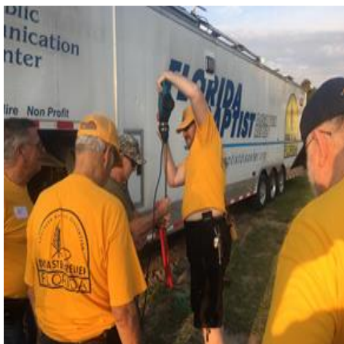
Electric Hammer Dill makes short work of ground rod installation
